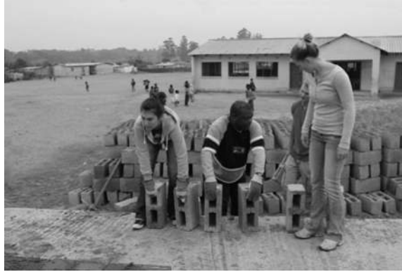
Moving Bricks Closer to the Foundations
