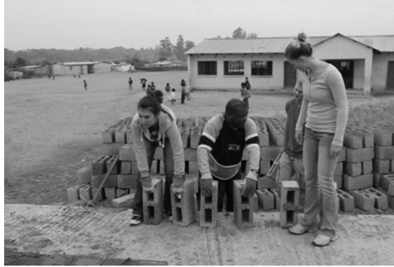
Moving Bricks Closer to the Foundations
