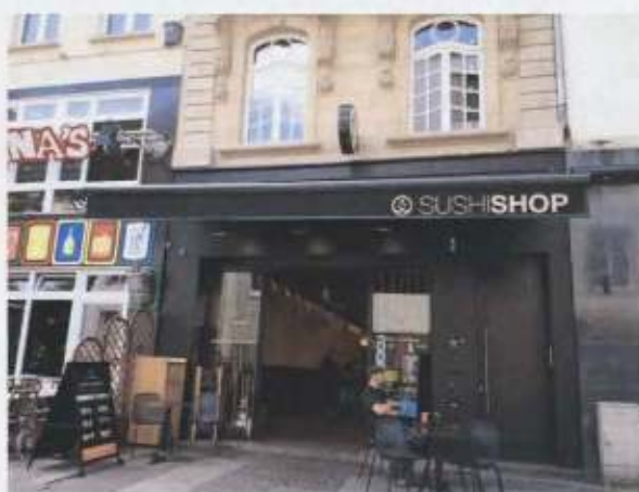
Figure 11– exterior of the Sushi Shop, an investigated restaurant
